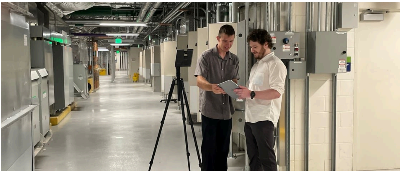
FIG. 2 – SMS TECHNICIANS VERIFYING CAPTURE COVERAGE ON SITE BEFORE LEAVING THE FACILITY.
